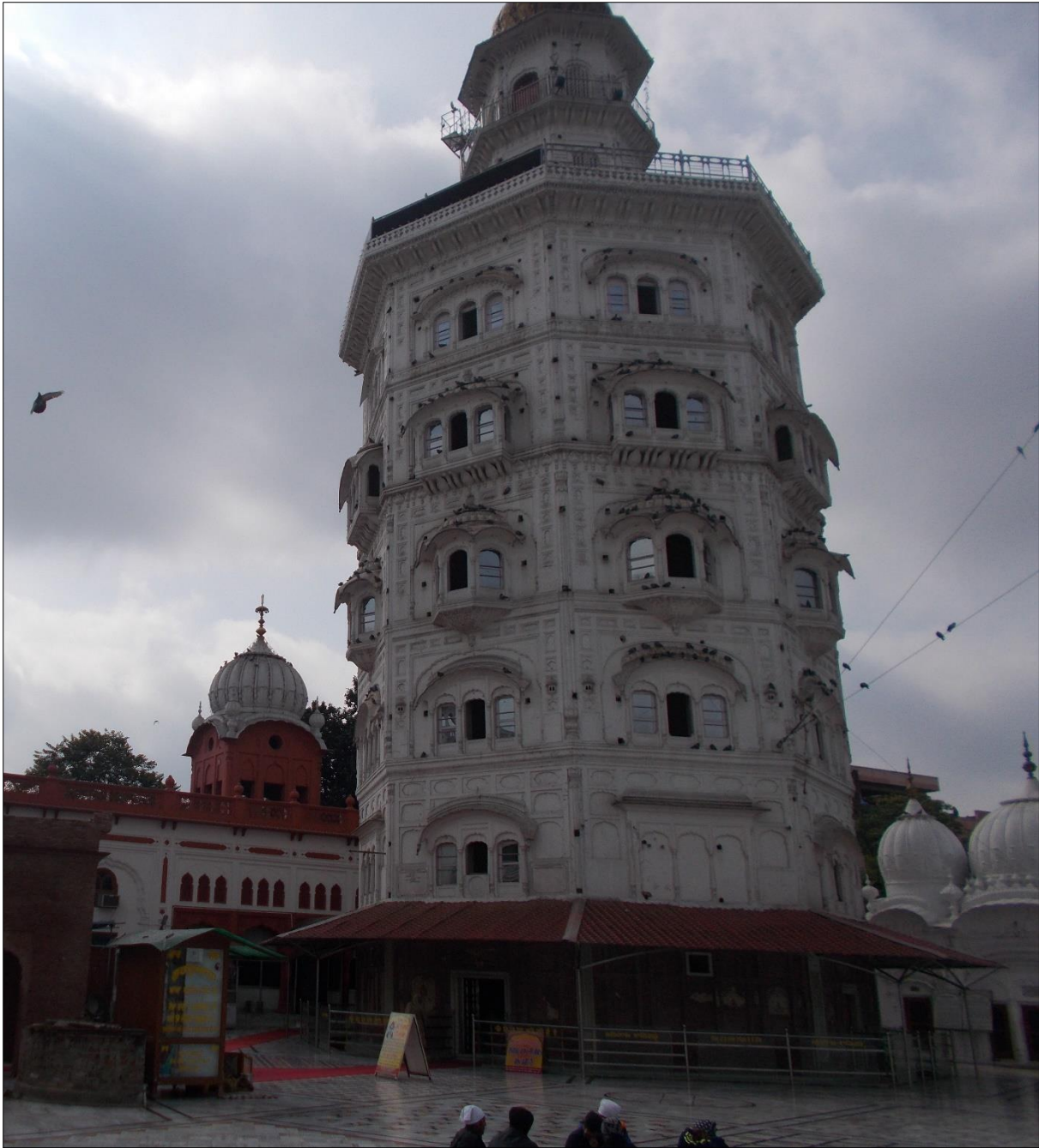
Figure 12: The Gurudwara Baba Atal Sahib Ji in Amritsar is a seven-storey building with several murals devoted to Guru Nanak's life on the inner wall of the First Floor (photograph: R.C. Kapoor, March 2017).
