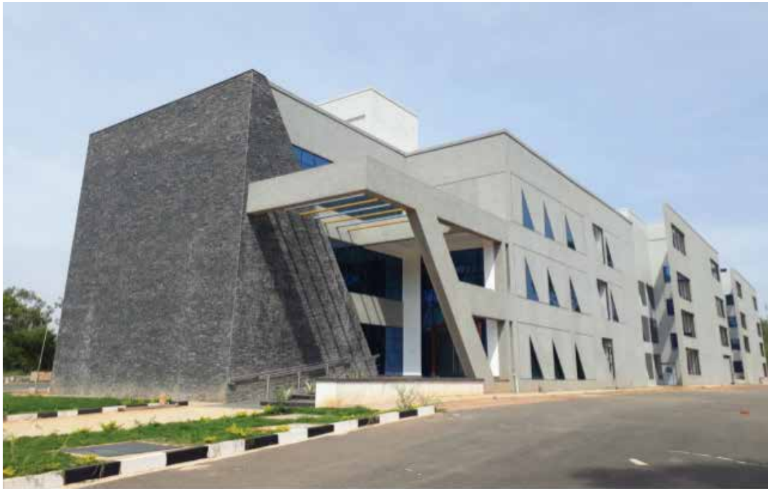
Figure 5.1: The ITOFF facility coming up at the CREST campus, Hosakote.
