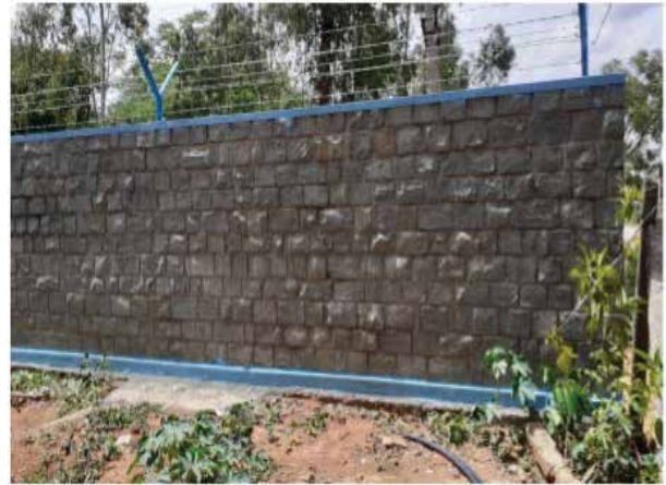
Figure 4.3: Stone wall construction around the CREST campus at Hosakote.
