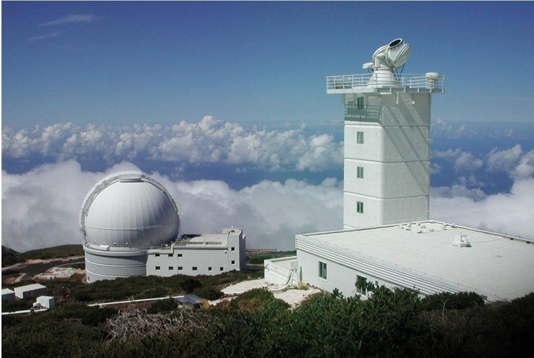
FIGURE 2.1: The Swedish 1-meter Solar Telescope (SST) at La Palma, Spain. The visible tower hides a vacuum tube over which the primary of 1-meter fused silica lens is placed which converges the solar light at the base and form an image. Image credit: https://www.mn.uio.no
