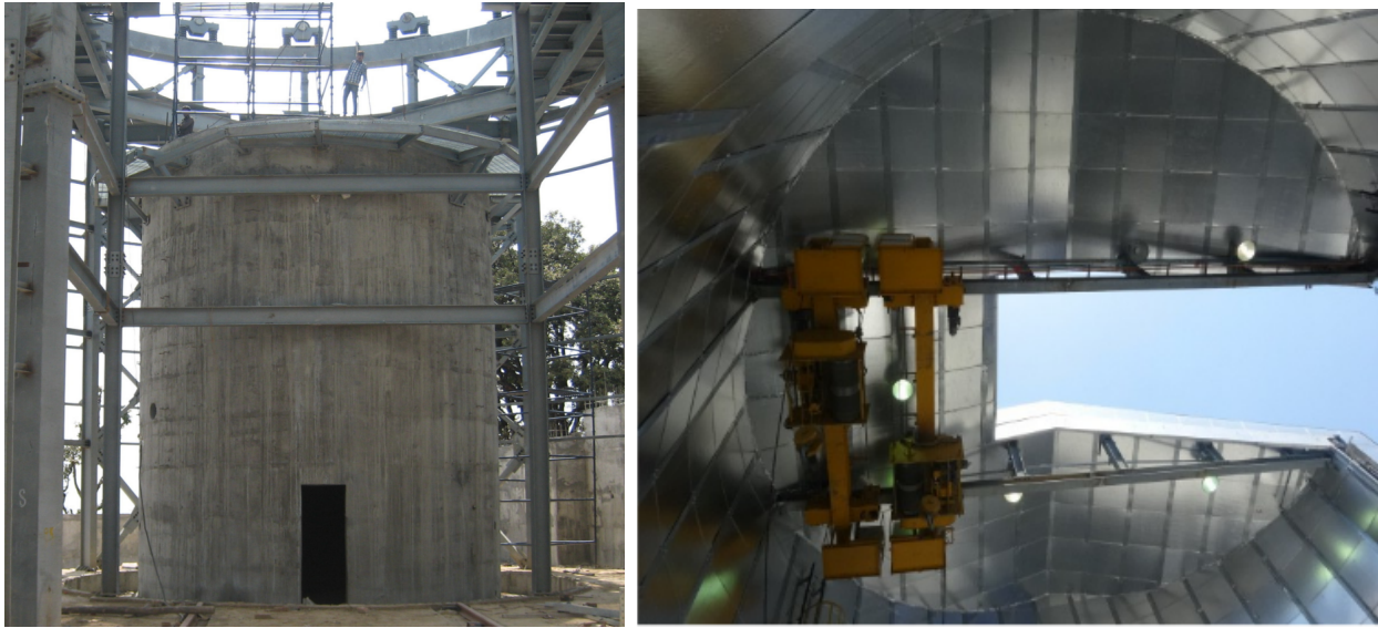
Figure 5: Left: A picture of the 3.6-m telescope pier. The pier is a hollow cylinder with an inner diameter of 5 m, an outer diameter of 7 m, and a top slab with a thickness of 1 m. The height of the pier from the ground is 8.26 m. Right: A picture of the dome overhead cranes.
