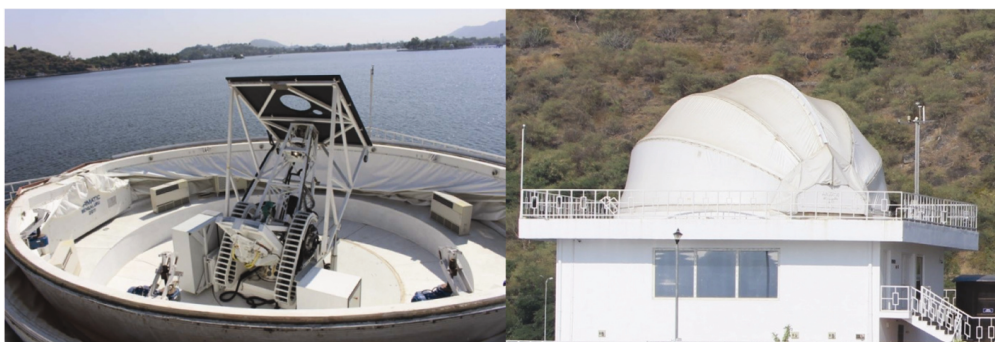
Figure 3. The telescope enclosed in a dome made of tensile cloth. (Left) Dome opened for observations, (Right) Dome in the closed position.
