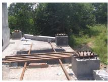
Figure 2.10: left: Determining the true N-S centerline on the top slab of the pier (May 2011). center: Completed pier and ground floor (September 2011). right: grouting of base plates for erection of steel building and dome at right (December 2011)
