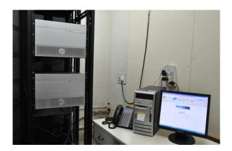
Figure 2.20: The IP based EPABX.
