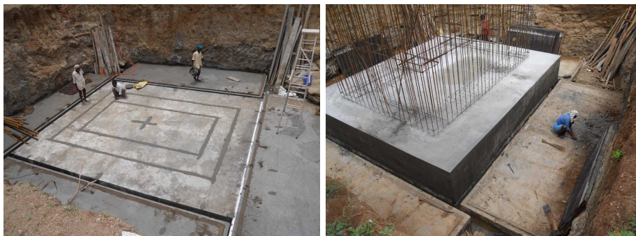
Figure 2.13: Casting of base of the Pier as in August – September 2010
