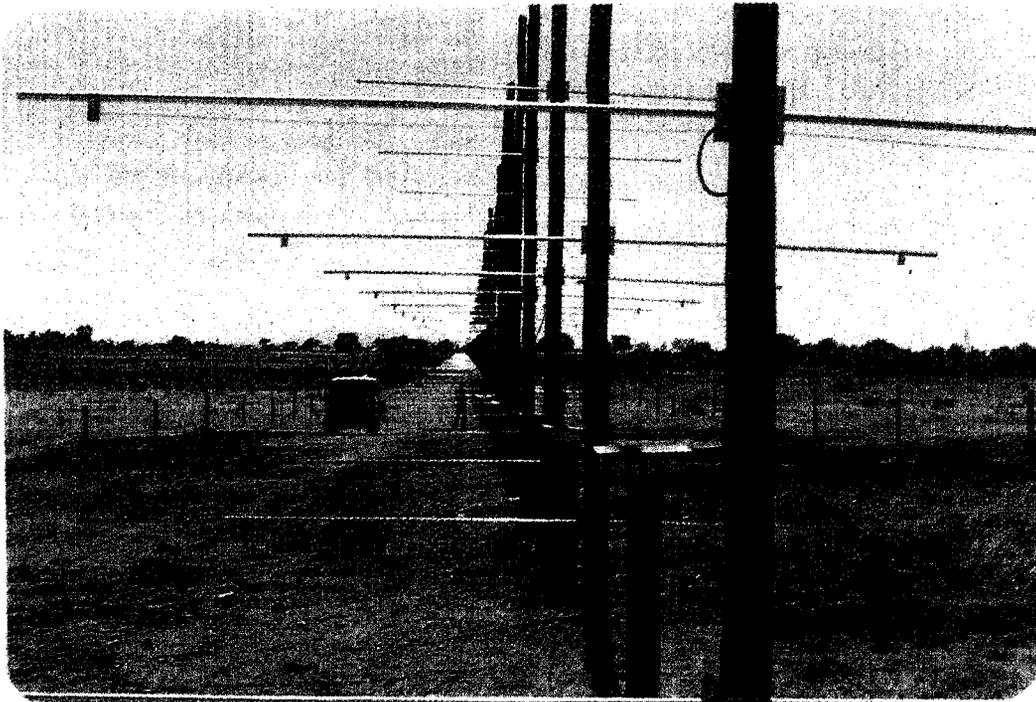
The northern arm of the Decametre Wave Radio Telescope at Gauribidanur
