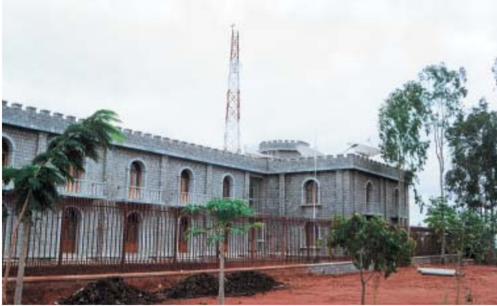
Remote control and data acquisition centre, Hosakote
