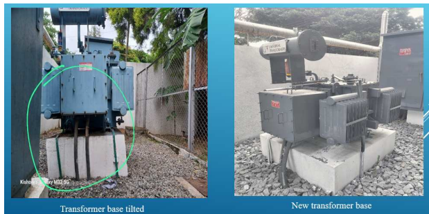
Figure 6.31: New Transformer Base
