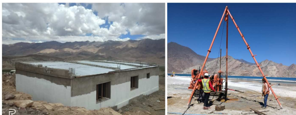
Figure 6.29: Civil Work at IAO, Hanle
