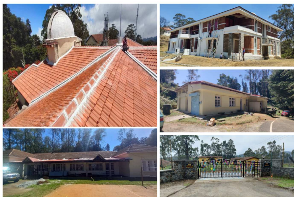
Figure 6.28: Civil Work at Kodaikanal Solar Observatory
