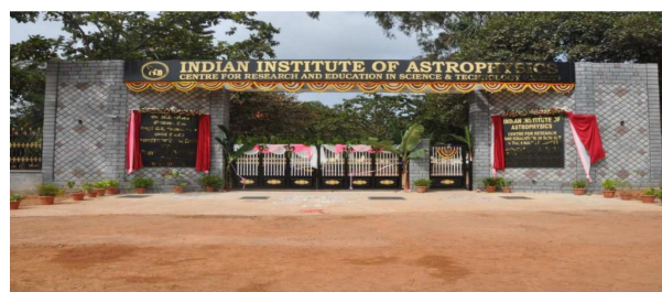
Figure 6.26: Civil Work at CREST Campus, Hosakote
