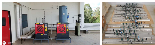
Figure 4.18: Left: Compressed gas generation & storage; Right: compressed gas distribution & controls at ITOFF.
