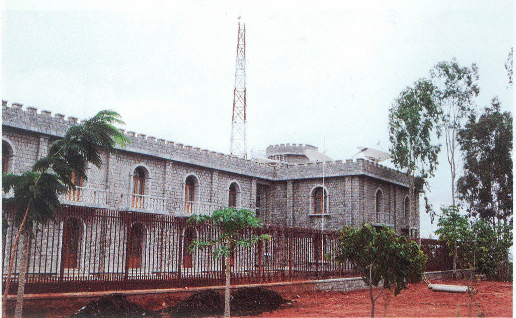
Remote control and data acquisition centre, Hosakote
