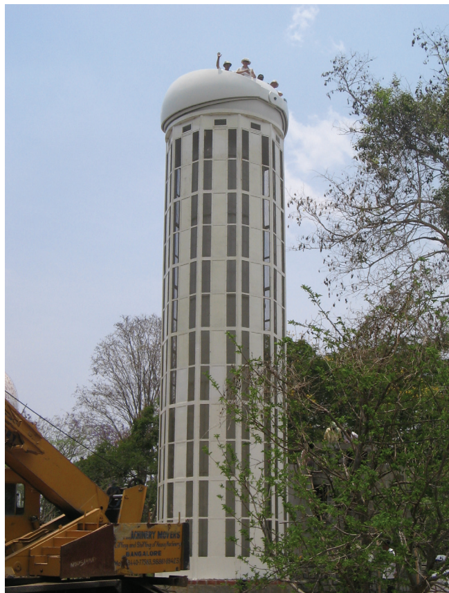
A happy team on top of the installed DIMM telescope tower and dome
