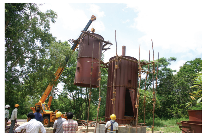
Installing the DIMM telescope tower at the Vainu Bappu Observatory
