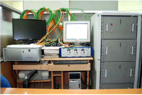
Figure 2.9: Control system testing.
