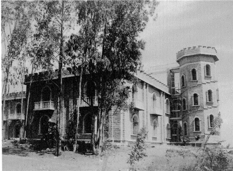
Remote control and data acquisition centre at Hosakote
