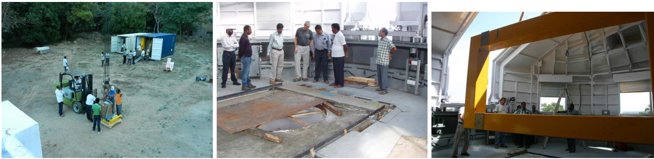
Figure 3.7: (left) Lifting out telescope parts from containers 7th February. (middle) Fixing the sole plates on top of the pier 11th February. (right) The base frame was lifted into the dome on 13th February.
