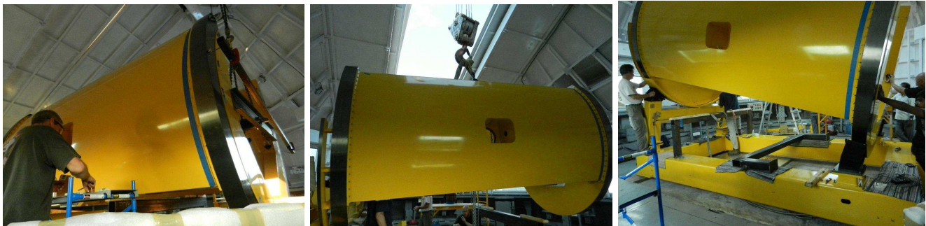
Figure 3.9: (left) Alignment tool mounted on the polar axis at south horseshoe. (middle) Assembled horseshoe mount held up by the external crane prior to positioning on the hydrostatic pads. The tool was for checking perpendicularity of the bearing surface. (right) Mount structure being positioned on bearing pads 18th February.
