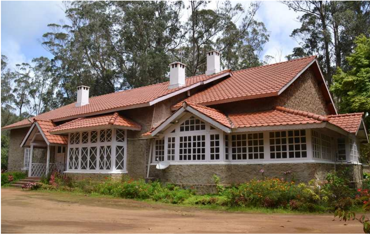
The Evershed Hall after renovation.
