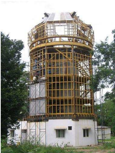
Figure 3.2: Steel building and dome structure (August 2012).
