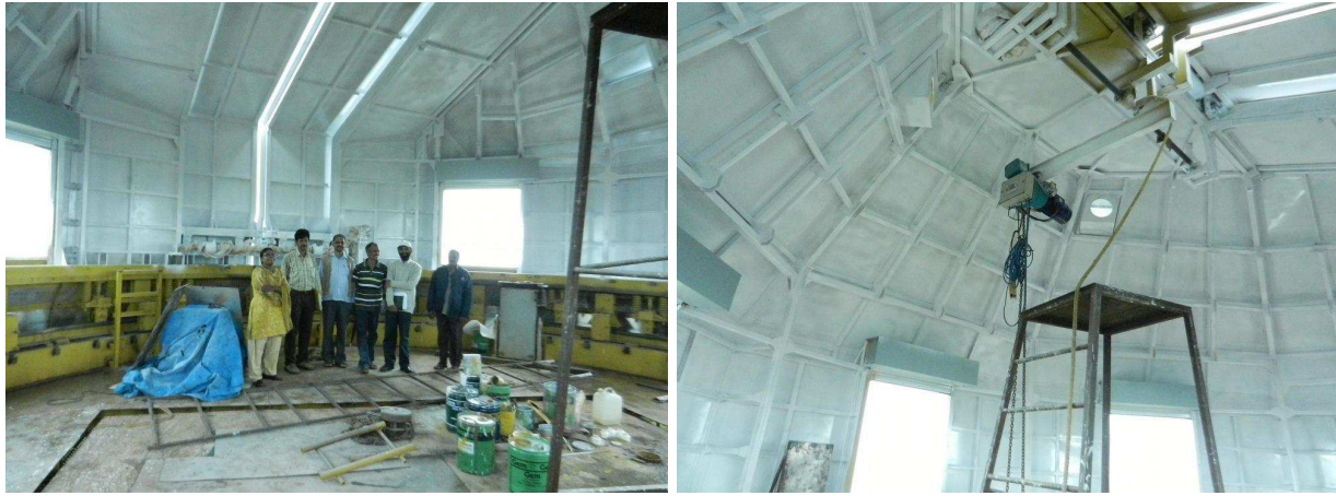
Figure 3.4: (left) Inside of the dome (Dec. 2012). One of the dome friction drive wheels is seen on the right. The top of the rectangular telescope pier is in the foreground. Some of the dome wheels and the rail are also seen. (right) The dome hoist of capacity 2 tons will be used for lifting the mirror cell through an opening in the top of the hollow pier.
