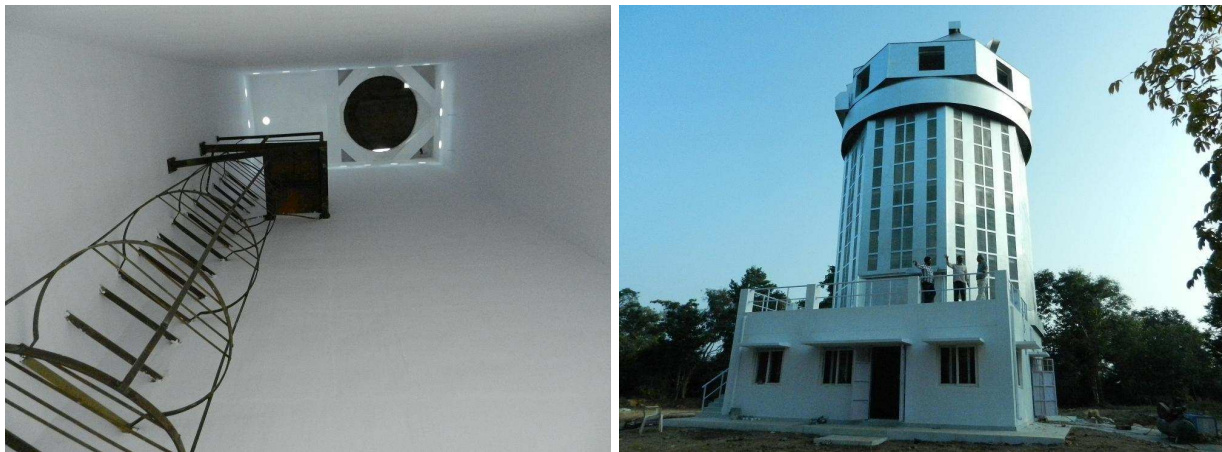
Figure 3.5: (left) Inside the hollow pier looking upwards. The ladder structure and platform is for installation and maintenance of the oil lines for the hydrostatic bearings of the telescope. The hole at the top of the pier is for lifting or lowering of the mirror cell from ground level. (right) The building/dome after painting in January 2013.
