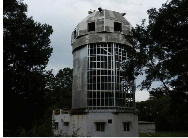
Figure 3.3: Aluminium cladding work on building and dome (October 2012).
