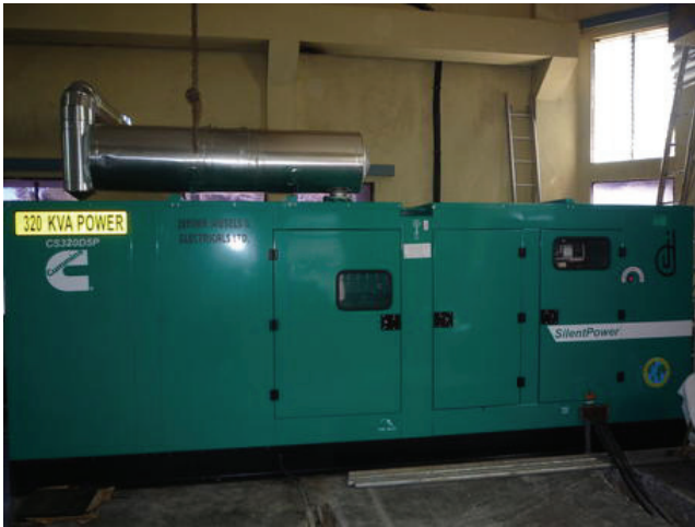
New 320 KVA DG set installed in Power House , VBO, Kavalur.
